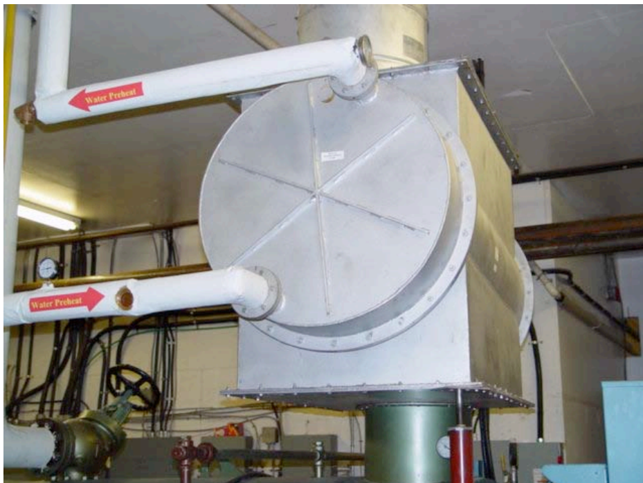
Figure 1 - Simple installation of Econotherm® GW unit
